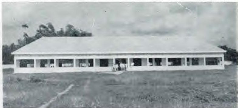
The rear view of the new Vietnam Training School is shown here to give an idea of the overall size of the school. See language section for other views.
