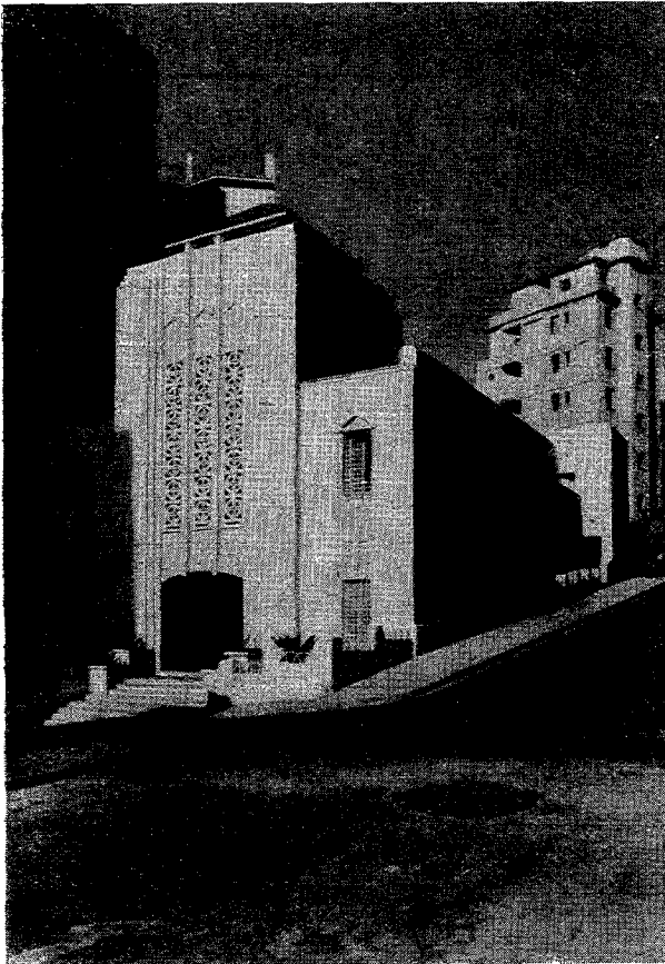
Chapel and union headquarters at Algiers.
