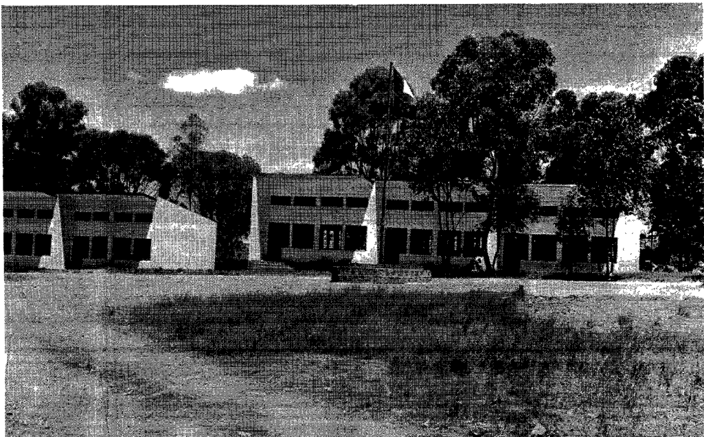
Two new school buildings at the Soamanandrarinny Seminary.
