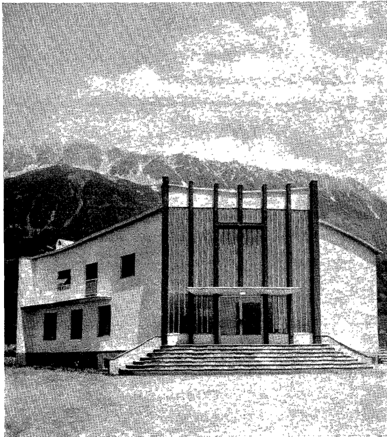
The new church in Innsbruck, Austria
