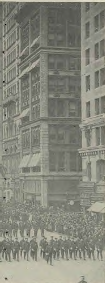
ing a part of the skyscraper section of ty.
