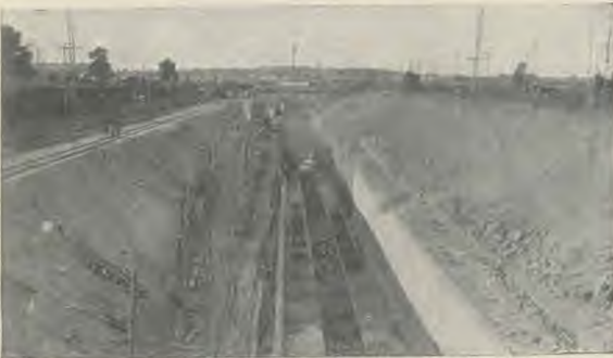
Section of Chippawa Canal
