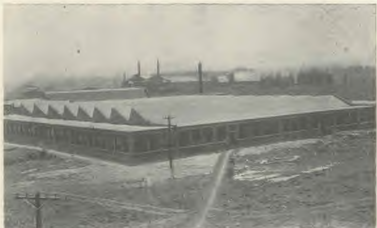
New Factory of The Imperial Steel Co., Collingwood, Ont.
