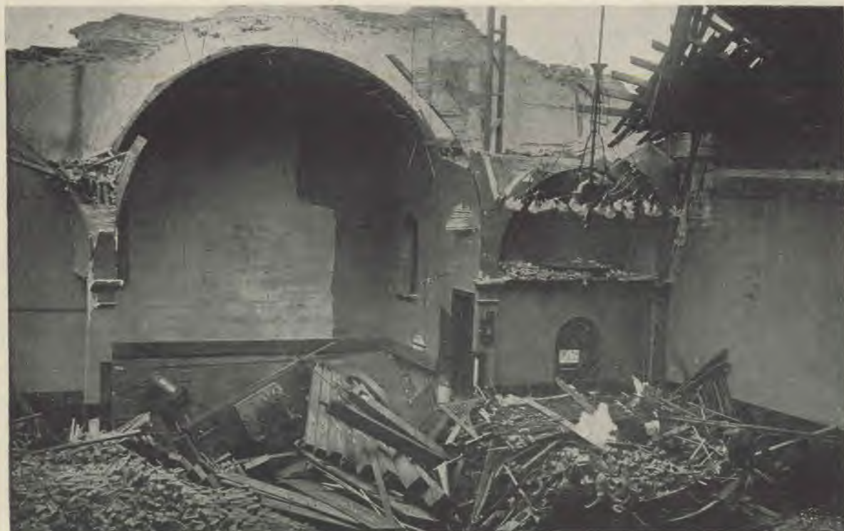
Ruins of a Church Building Destroyed by a Tornado at Portage la Prairie, Man., in June, 1922
