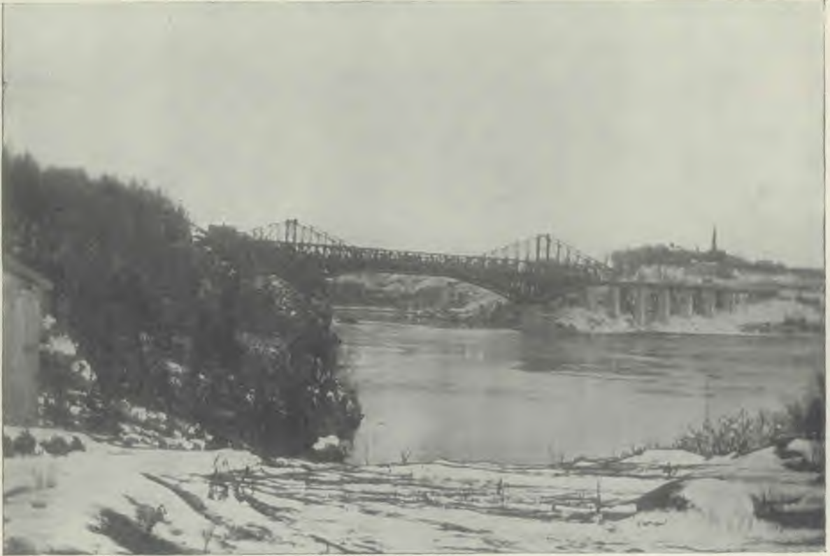
The New C. P. R. Bridge over the Famous Reversing Falls at St. John, N. B.
