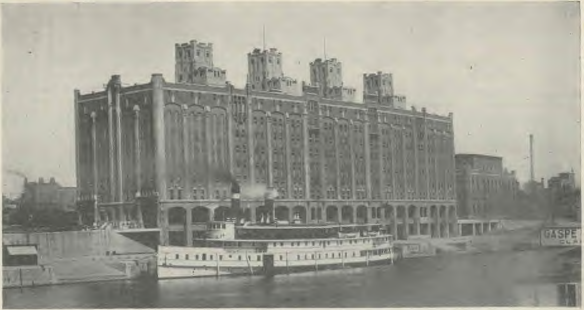
Warehouse and cold storage plant, Montreal. Dimensions, 440 feet by 110 feet; ten storeys high; storage capacity 4,628,000 cubic feet. An artesian well 1,100 feet deep supplies pure water of a temperature of 42° in summer. A feature of the equipment is the ice-making machinery.
