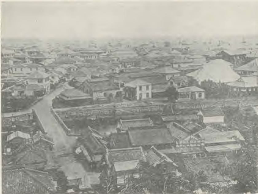
Yokohama as it looked before the earthquake. The city was almost entirely destroyed.
