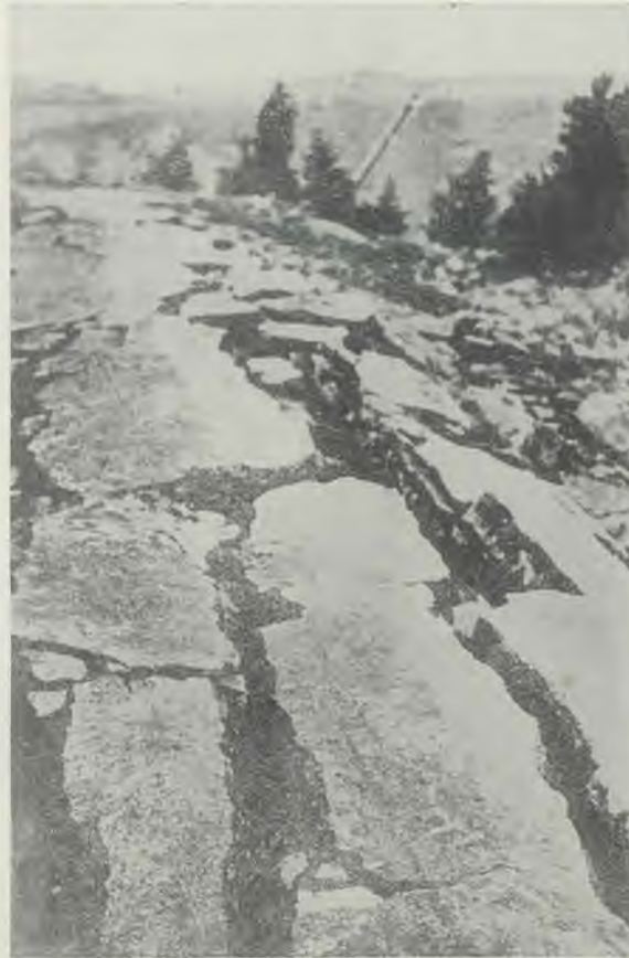
THE JAPANESE EARTHQUAKE Cracks in the earth's crust as seen at many points in the zone of destruction.
