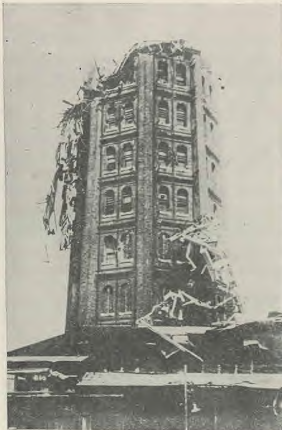
THE JAPANESE EARTHQUAKE Remains of a thirteen-storey building in Yokohama, which cracked from the seventh floor upward.
