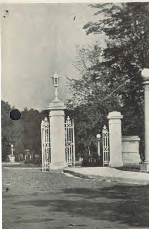
to, showing the new ornamental iron gates nted with lanterns
