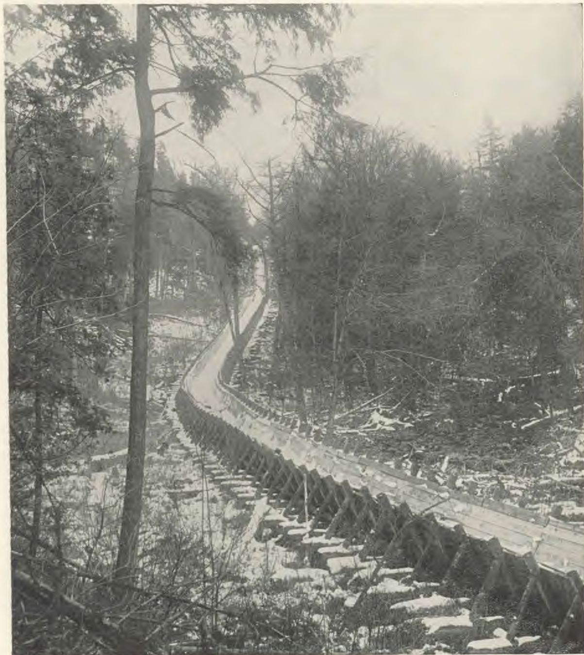
A TIMBER CHUTE
