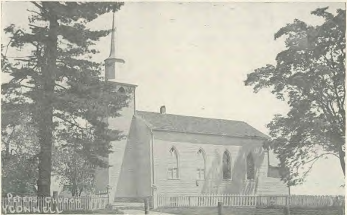
St. Peter's Church at Tyrconnell, near St. Thomas, Ontario, erected nearly one hundred years ago.
