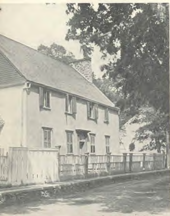
Old Store, Quebec, which dates from 1637. Buildings in Canada.
