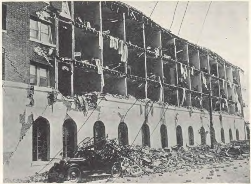
When the earth shuddered. The photograph shows the hotel California, in Santa Barbara, with an outside wall stripped by a peculiar prank of the earthquake, exposing the rooms. Several of the guests were killed, while others were not even awakened by the quake.
