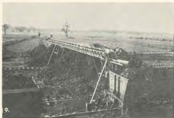
Right — Conveyor and storage yard of prepared fuel peat, at Alfred, Ontario.
