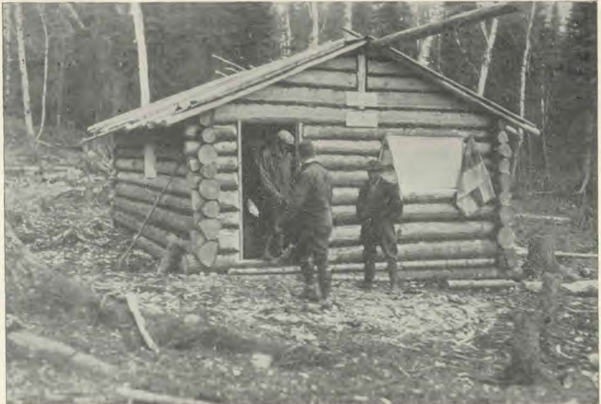
Post office at Red Lake mining camp. Note the background of heavy timber.
