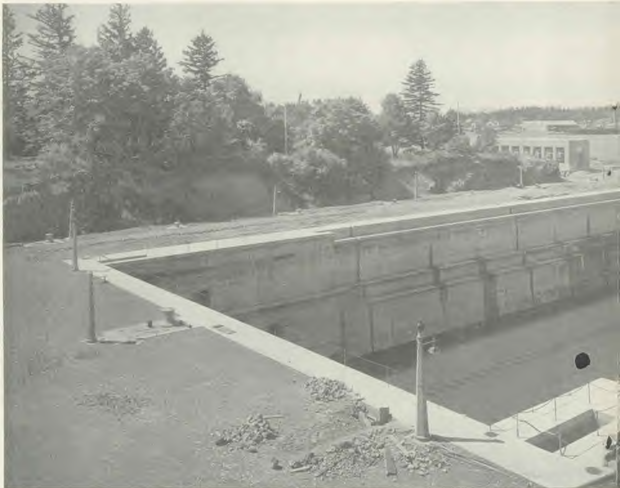
The great new drydock at Victoria, B. C. The naval barracks and the Harbour of Esquimalt in the background. It is the largest in the world, with a length of 1171 feet. There are now fourteen drydocks in the world having a length of 1050 feet.
