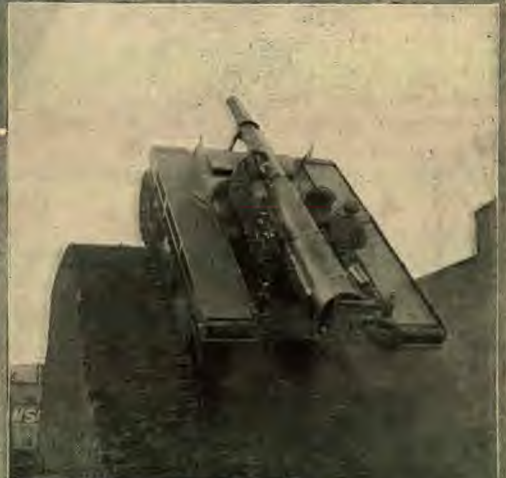
Left: A new 16-inch disappearing gun with bomb-proof shelter that throws a 2,700-pound shell 35 miles and weighs 510 tons.
