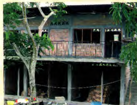
The top three rooms of the Crisis Center Dormitory are almost finished, and the bottom floor is well under way. Twelve more rooms are in the plans for this complex.
