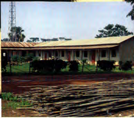
UNIFAT School before the construction of the fence.
