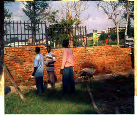
UNIFAT's partially completed fence
