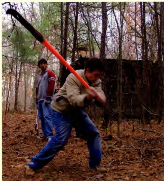
Outdoor leadership majors Sunny Tier and Casey Walter work on repairing old cabins.
