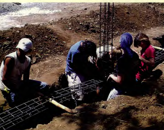
One project at the orphanage was to group rebar together by hand for the footers and columns of the maintenance building, in preparation for pouring of the cement.
