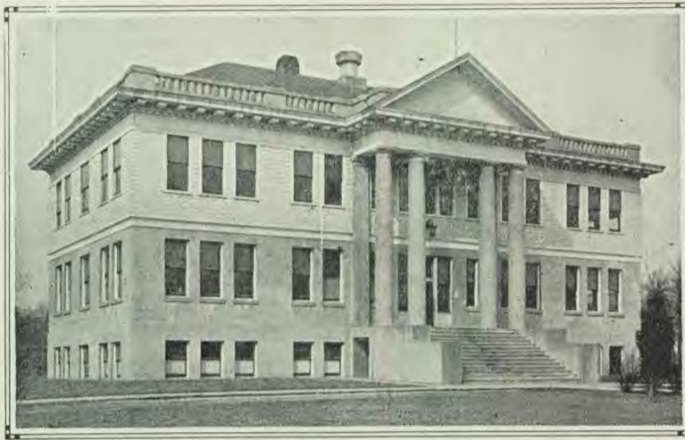
College Hall, W. M. C.'s first Administration Building and now the home of Science and Normal Departments
