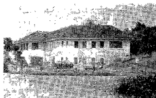
CAU's headquarters office building, Bujumbura, Burundi.
