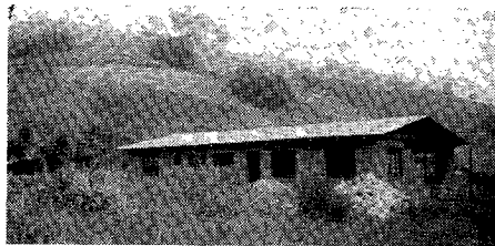
New house for an expatriate worker going up at Kivu Adventist Seminary.
