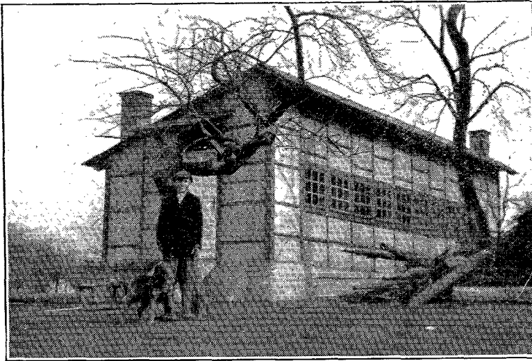
Carpenter's shop of the Polish Mission School, built by students, 1929.
