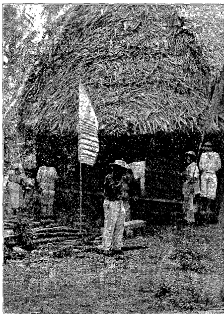
FINISHING A HOUSE.
