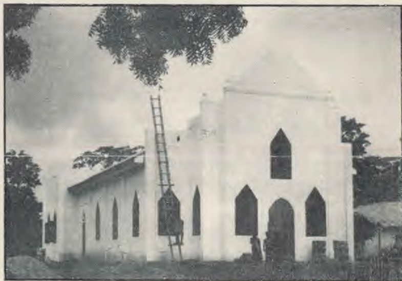
Beautiful new church built almost exclusively by the members at Ntonso Gold Coast. Well done members at Ntonso. God is pleased when we build a fine house to meet Him in.
