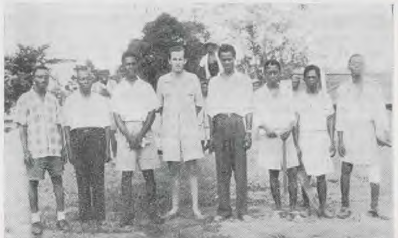
Picture from left to right: Mr. F.A.T. Fofana, Pastor J. S. Myers, Mr. Weston (Architect), Mr. J. Muderspach, Assistant Architect & Labourers, standing on the site of the new Bo Church.
