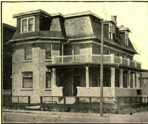
NEW HOME OF WESTERN CANADIAN TIDINGS
