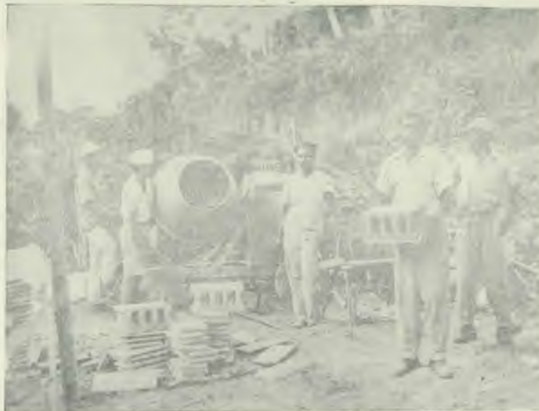
MAKING CEMENT BLOCKS
