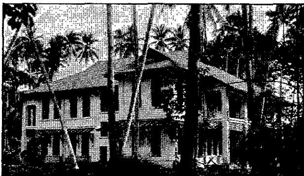
One of a group of buildings forming the Penang Mission Clinic in the Straits Settlements of Malaya. Our society gave the land, and a portion of the money, but the larger part of the expense of erecting the buildings has been borne by friends of the Mission Clinic.
