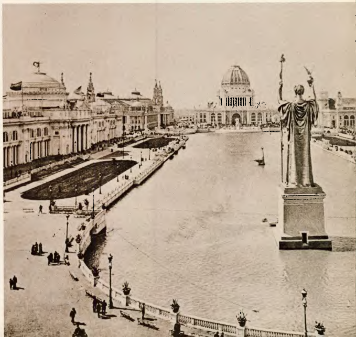
This view of the Grand Basin and Court of Honor shows the immensity of the construction.
