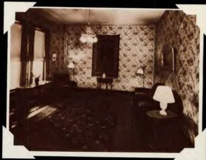
Lobby of old South Hall before the fire
