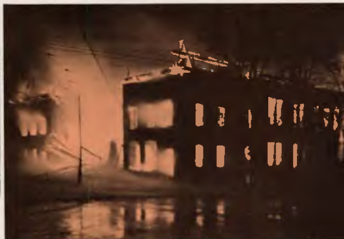
Fire totally demolished the publishing house on the evening of December 30, 1902.
