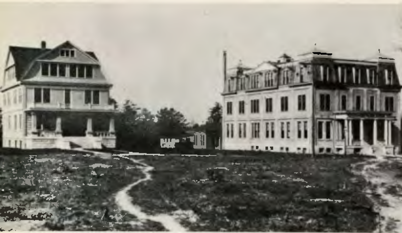
By December, 1905, the new General Conference building (left in photo) was ready for occupancy. The Review and Herald building, which was completed in 1906, is next to it. Both buildings, which were built on the Thornton Tract, are still in use though now encased in numerous additions and covered with a brick facade.
