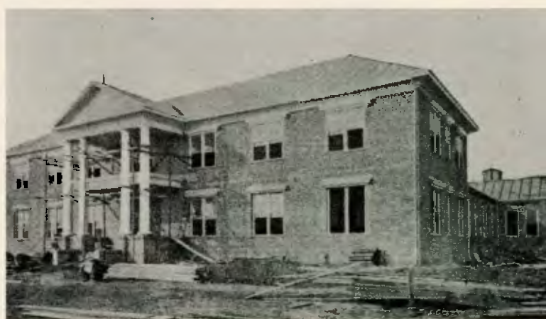
Press at Mountain View under construction, 1904 credit: Pacific P
