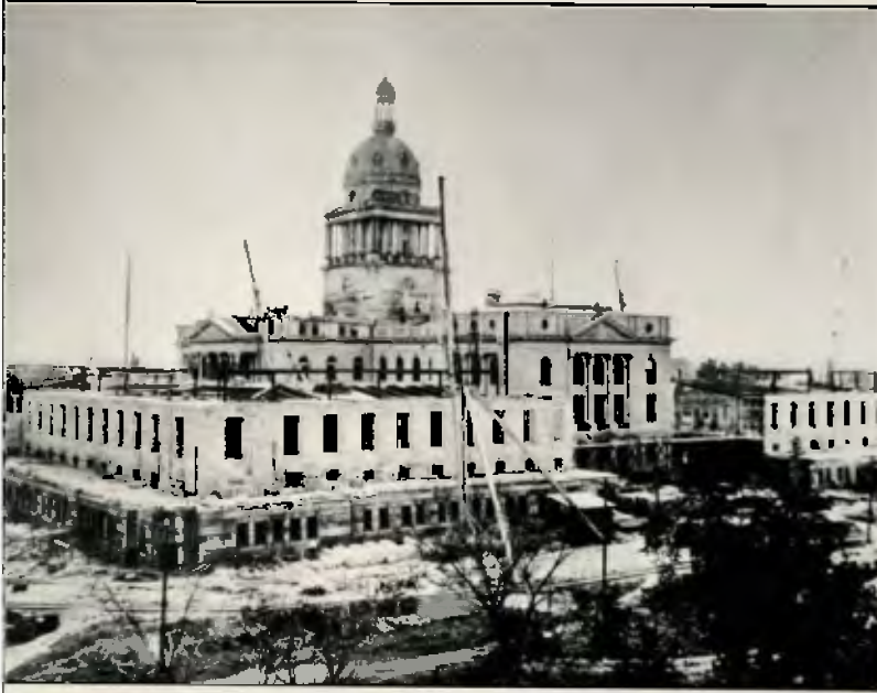
During Williams' terms as lieutenant governor of Nebraska, the third state capitol was constructed around the second building. The original one was eventually demolished as work on the new building progressed.
