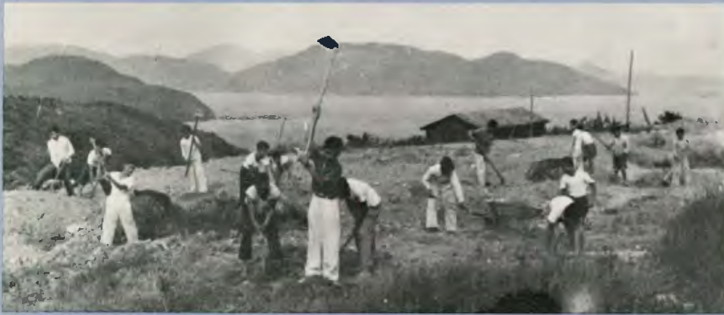
Students helping to clear the grounds at Clear Water Bay, prior to erection of the new buildings.
