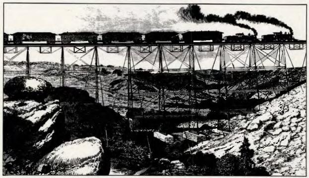
The largest trestle on the Union Pacific carried trains across Dale Creek just west of Sherman, Wyoming. This frail-looking iron structure replaced an earlier wooden bridge in 1876. It was dubbed "The Spider Web."
