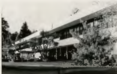
W.J. Blake Administration Building (1969)
