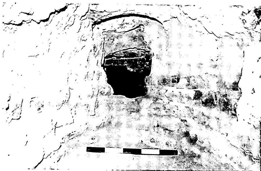
B. The inside of the furnace looking toward the horizontal flue which begins at the hole in the background. It heats the bathing room above. The edge of a black basalt slab is visible on which the floor tiles rest. Photo: Avery V. Dick.
