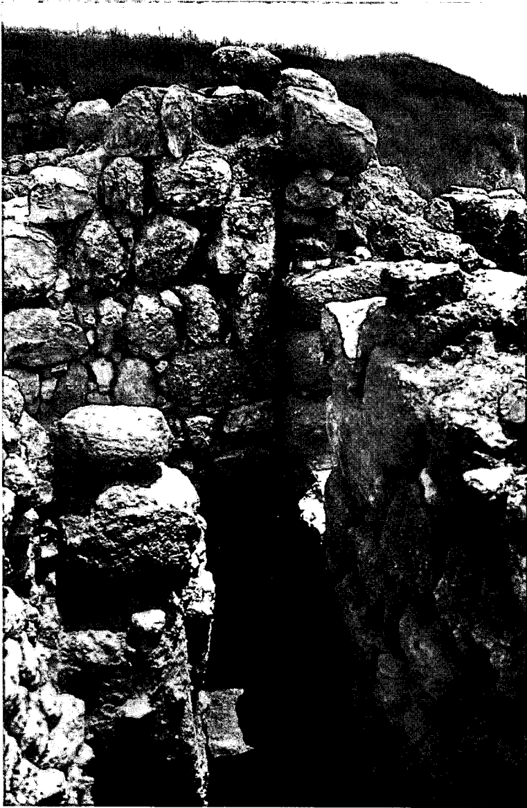
Plate 9. Join of the gate complex (left) and casemate wall (right).
