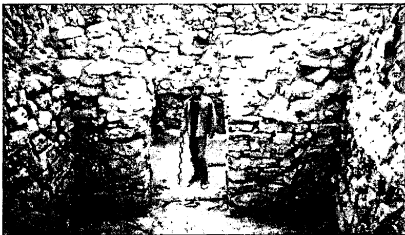
Figure 7. Tall al-'Umayri: Looking from the western room of the LB building in Field B through the door, illustrating the excellent masonry and preservation of the walls. The upper courses were consolidated with cement in 1998 to protect the walls from destruction.
